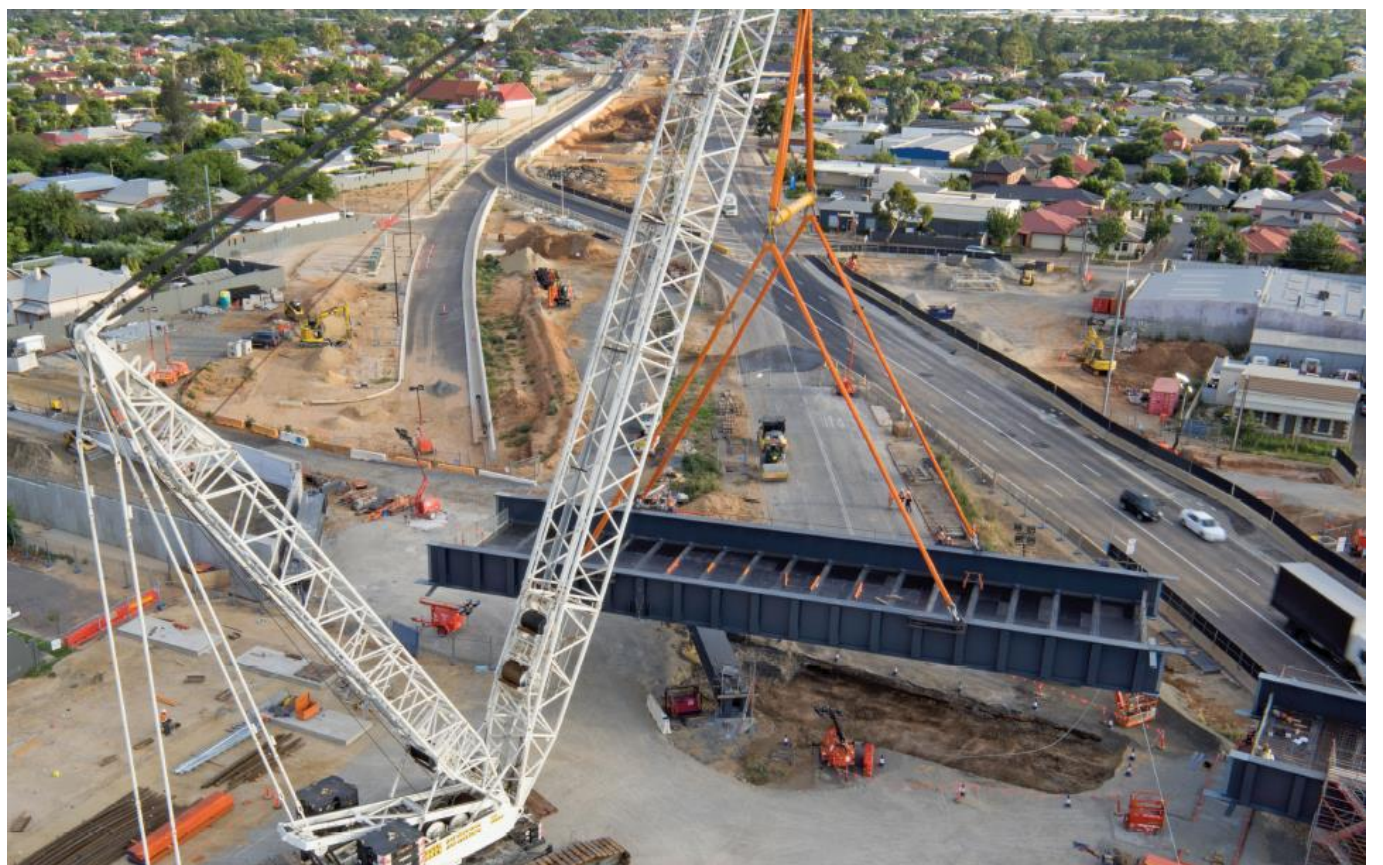
Installation of segment 2 of the Outer Harbor rail bridge
